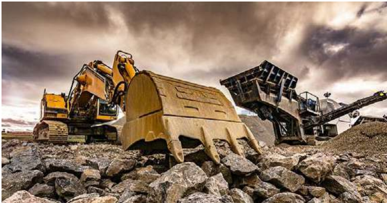
Plant Machinery & Vehicles
