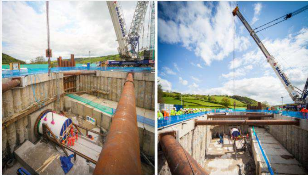
(left) By combining the tunnel drive pits and connection cofferdams, the team made significant savings while simplifying construction and reducing the delivery programme and (right) the three sections will bypass key locations of the aqueduct to improve resilience of water supply to Birmingham using this 100-year old asset - Courtesy of GHD
