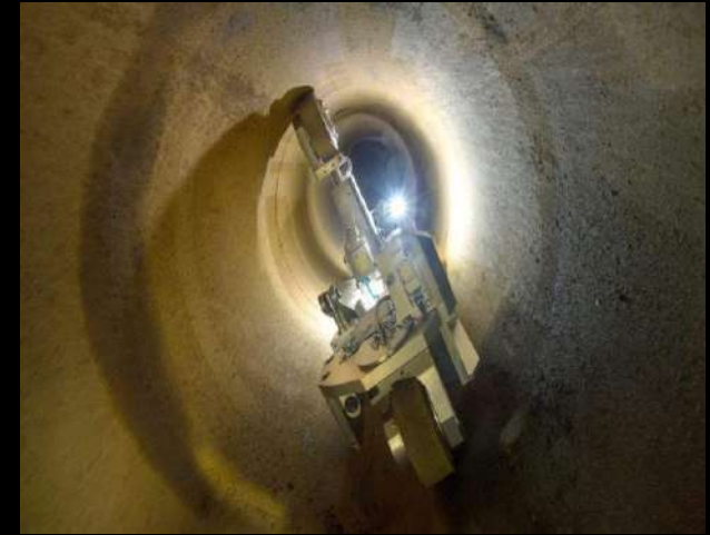
and in pipes
