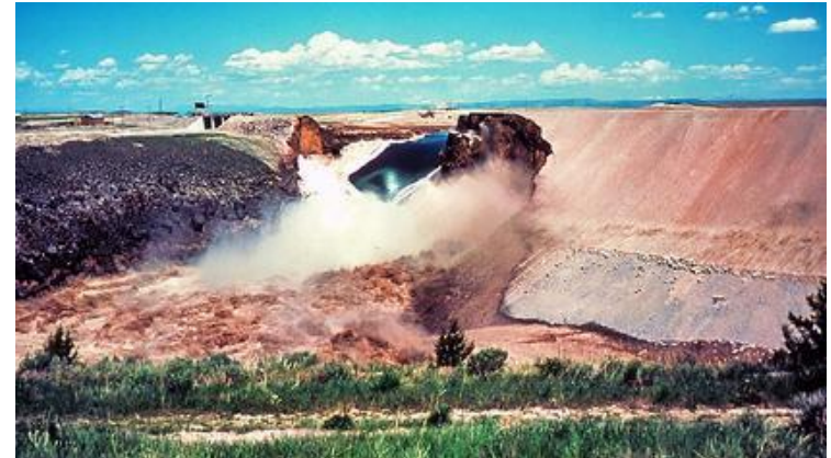
The collapse of Teton dam (Wikipedia)
